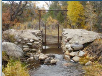
Acequia headgate (photo: Marcos Roybal)
