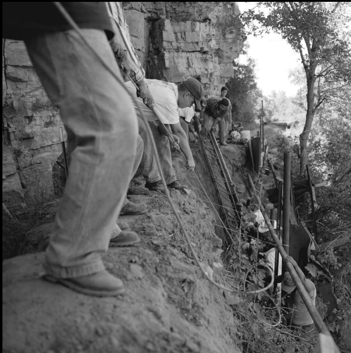
Ditch Repair at El Cerrito 1998
